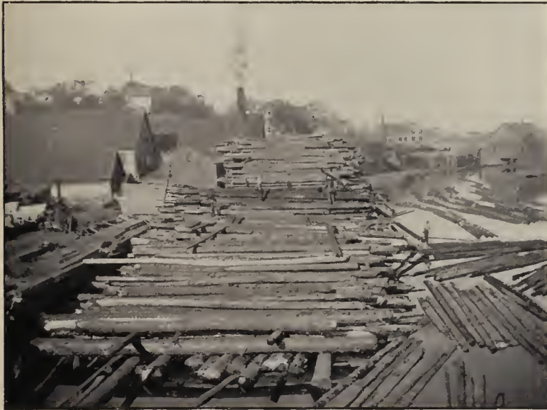
PILING LOGS AT J. GRAY & SON'S MILL.
